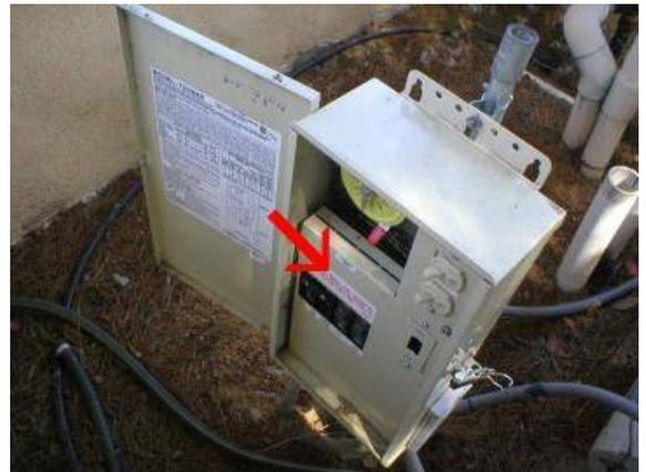
619 WORKMANSHIP The wiring within the panel appeared serviceable.
