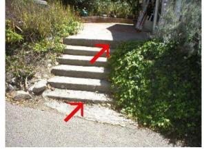
**222 HANDRAIL(S)** [SC] There are no handrails at the steps, required when 4 or more steps.
