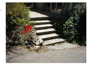
223 MAIN ENTRY [SC] Evidence of ponding water is noted on the entry porch. This condition is a slip and
